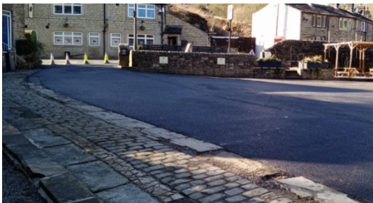
Resurfaced Turkey Inn Car Park
