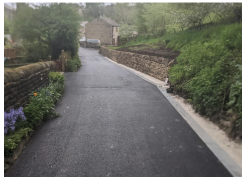
Lund Lane Resurfaced with flood channel installed
