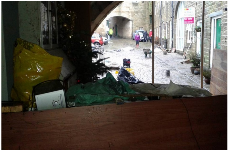
Flood Water destroys arch window in 2015 event.
