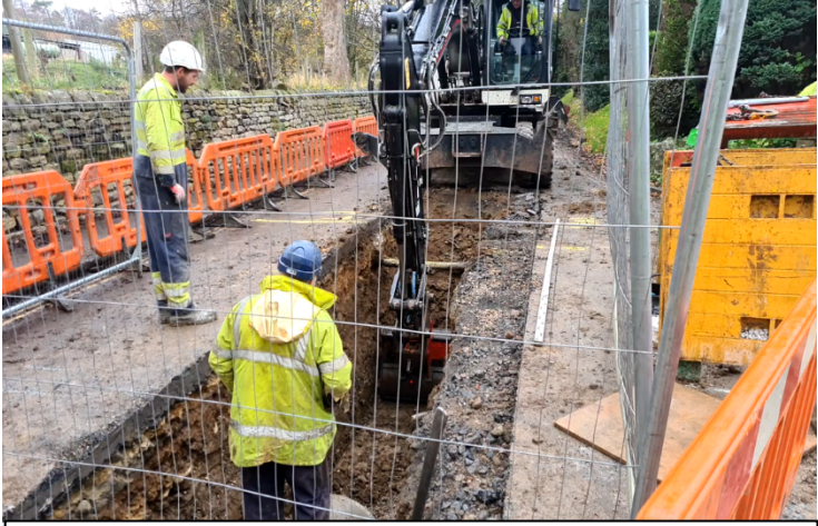
Restricted working room casued logistical challenges
